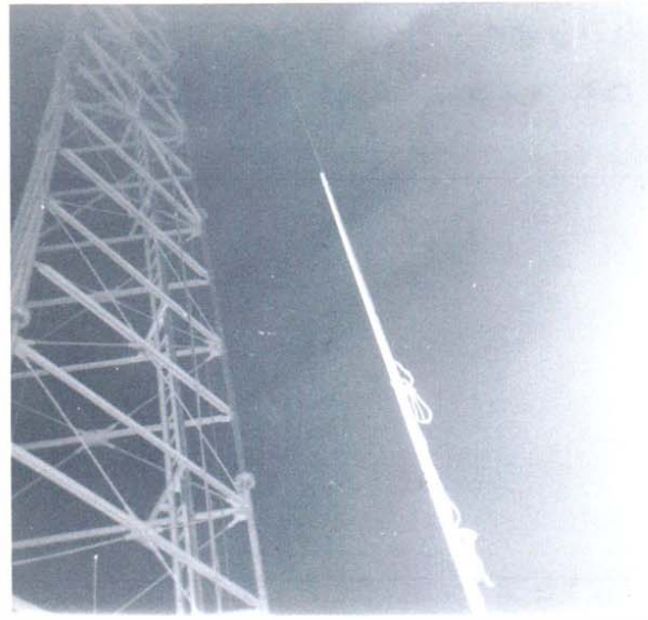
The antenna on its way up the tower.
